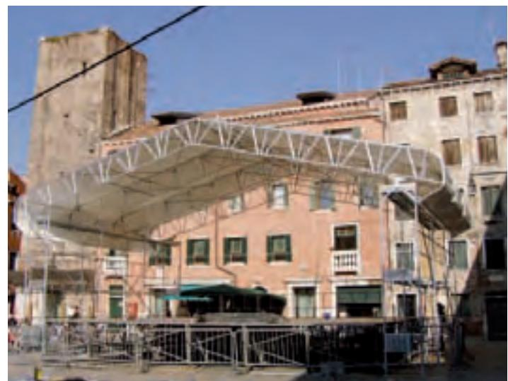
The beams which make up the main tie beams have a double "C" upper profile allowing rapid insertion into frames of 2.5 m. The polyester sheets, covered with PVC weighing 600g/m<sup>2</sup>, are of fire resistance Class II. They have flexible side stringing and are anti-freeze treated, allowing free movement along the beams.
