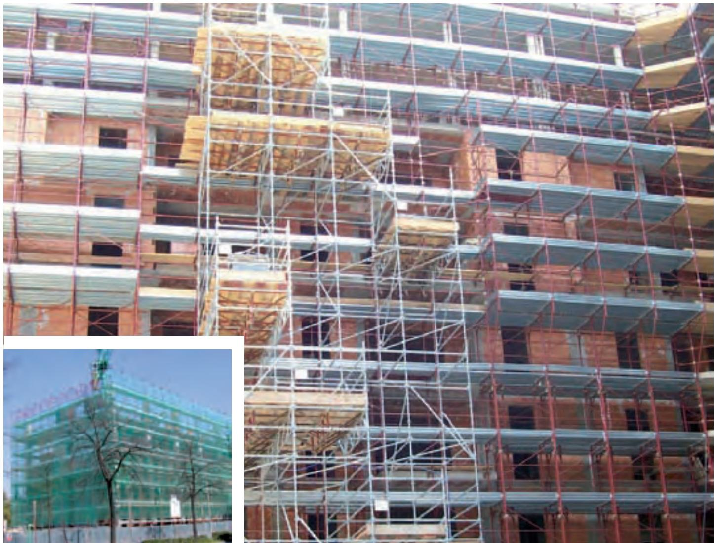
boards with trap door and stairway, side guardrails, gravel guard, guardrail post of 100 and 200 cm, galvanised adjustable base plate and aluminium guardrail to work in complete safety conditions during the assembly and disassembly phases. In addition, for the realization of the whole technical documentation to provide on each site, Pilosio S.p.A. made a software called MAS which allows to produce almost automatically CAD drawings in each view with the relevant list of equipment needed.
